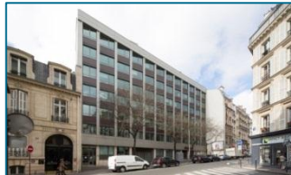
View of building after completion of renovation
