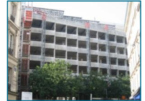
View of building during the heavy renovation works
