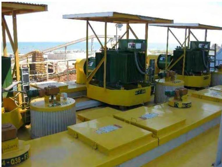
*Courtesy of ARAUCO Chile. Oil-Filled Transformer above the Electrostatic Precipitator*
