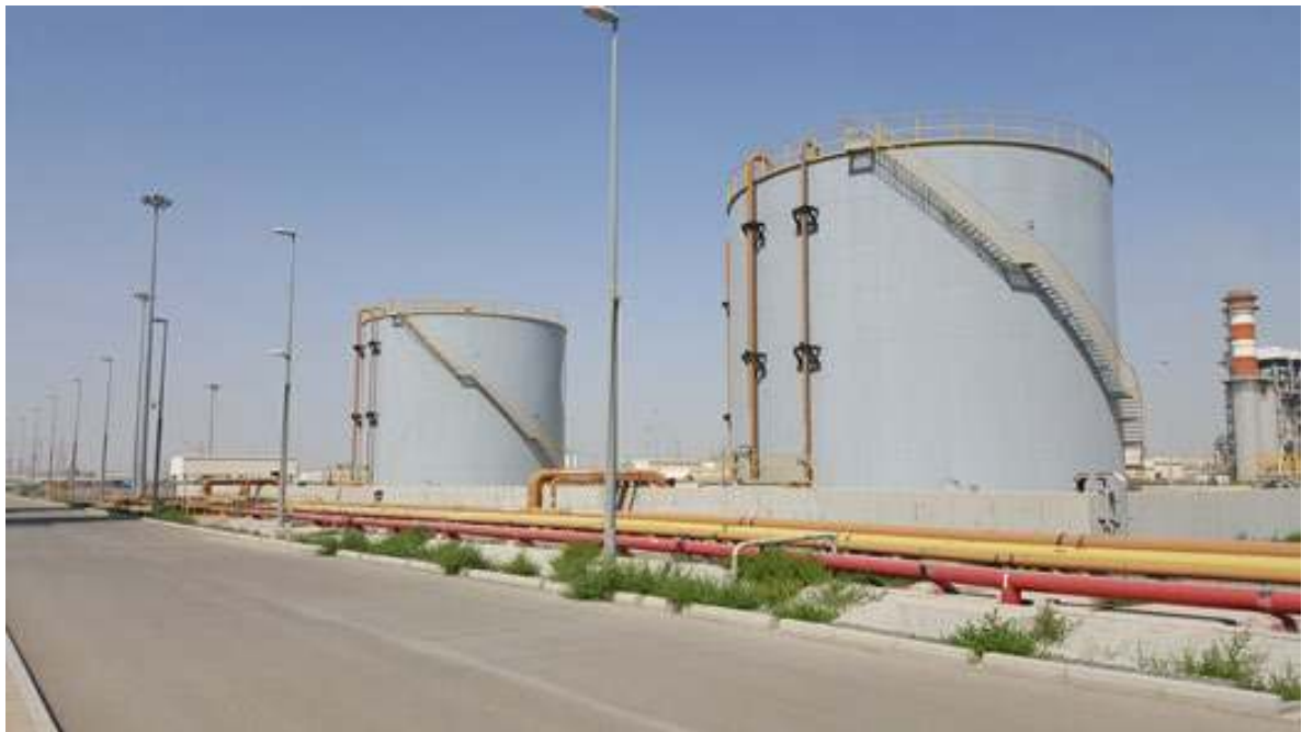
Fuel oil tanks adequately spaced and secondary retention provided Courtesy of SOHAR Aluminium LLC - Captive Power Plant
