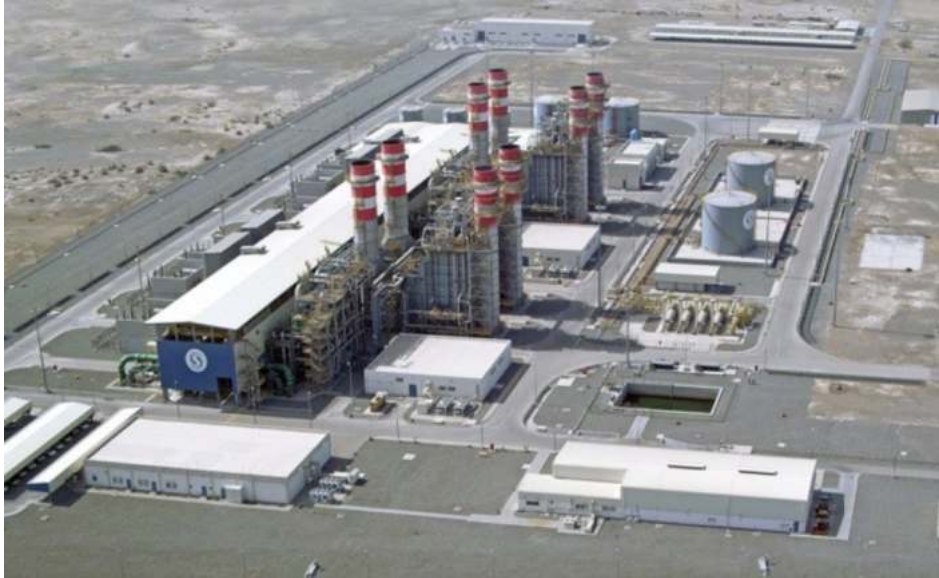
Captive Power Plant Courtesy of SOHAR Aluminium LLC
