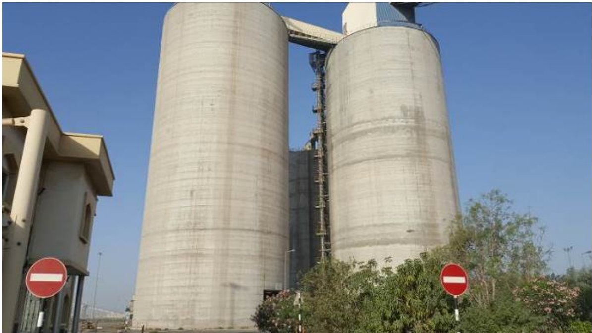
Alumina silos Courtesy of SOHAR Aluminium LLC
