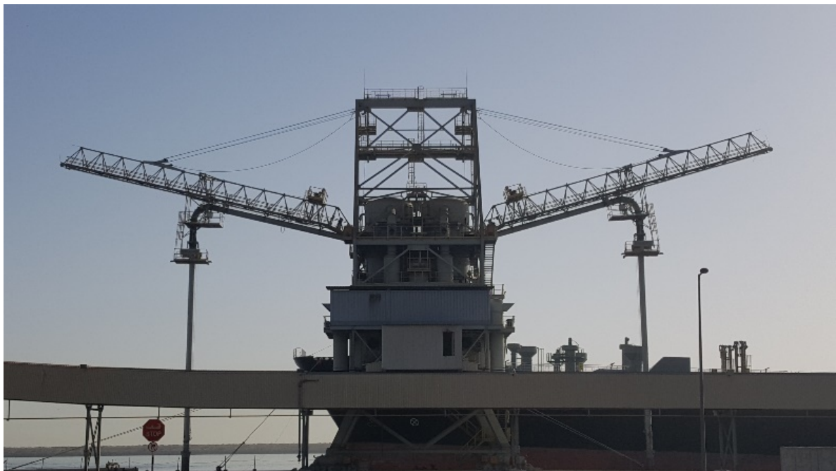
Coke & Alumina unloader Courtesy of SOHAR Aluminium LLC
