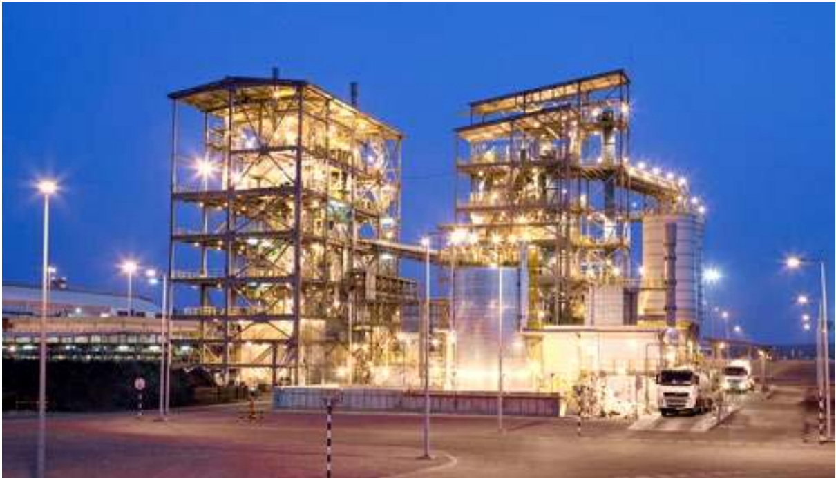
Carbon Plant – Sprinkler protected paste plant Courtesy of SOHAR Aluminium LLC
