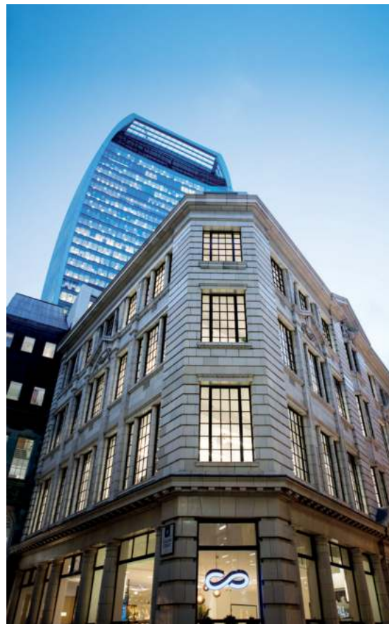
London office / United Kingdom - Certified BREEAM
