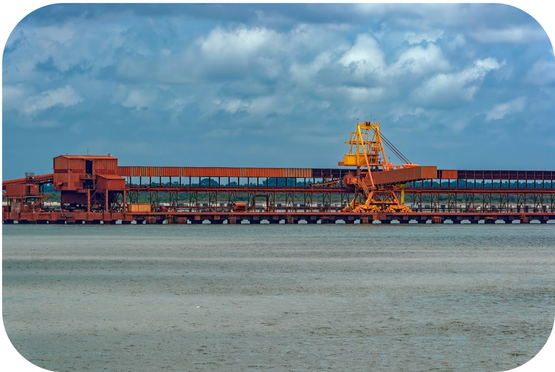
Bauxite conveyor from the stack to the loader
