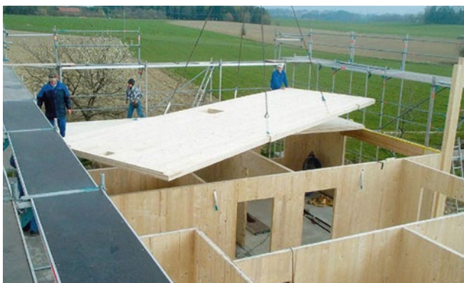
FIGURE 5 - PANNEAU MASSIF CONTRECOLLÉ OU CROSS LAMINATED TIMBER (CLT)
