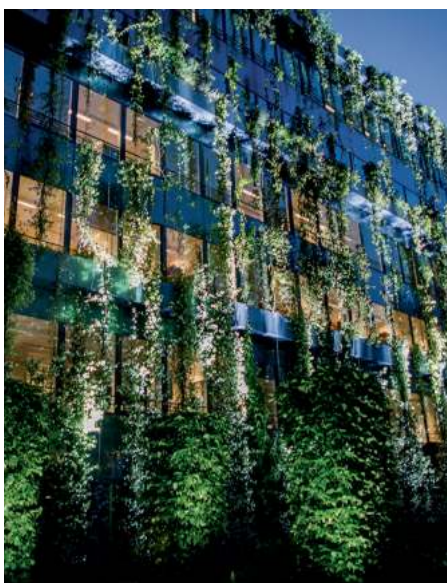
SCOR's Paris Headquarters, certified Haute Qualité Environnementale
