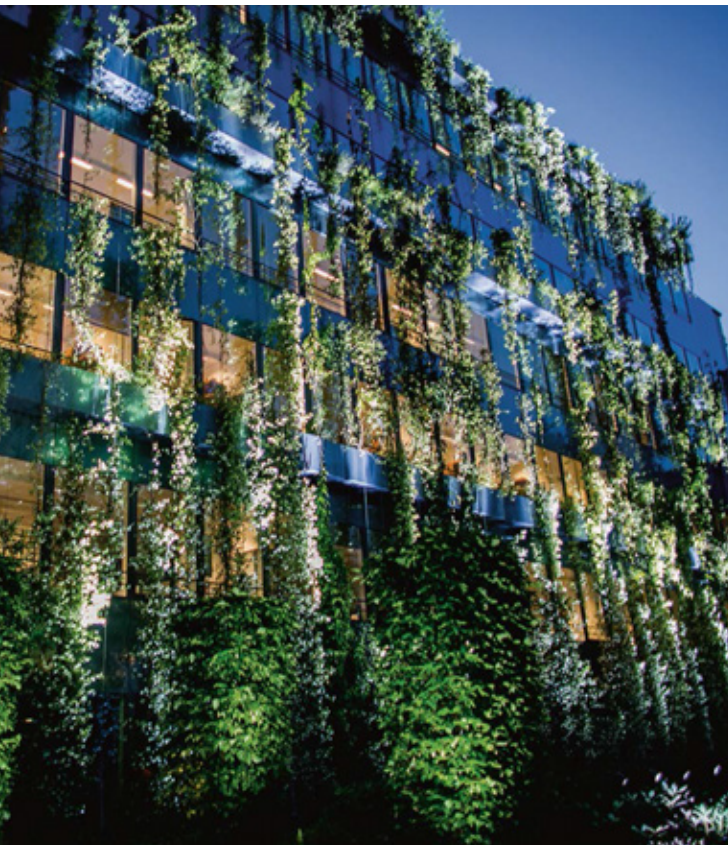
SCOR's Paris Headquarters, certified Haute Qualité Environnementale (high environmental quality) or HQE
