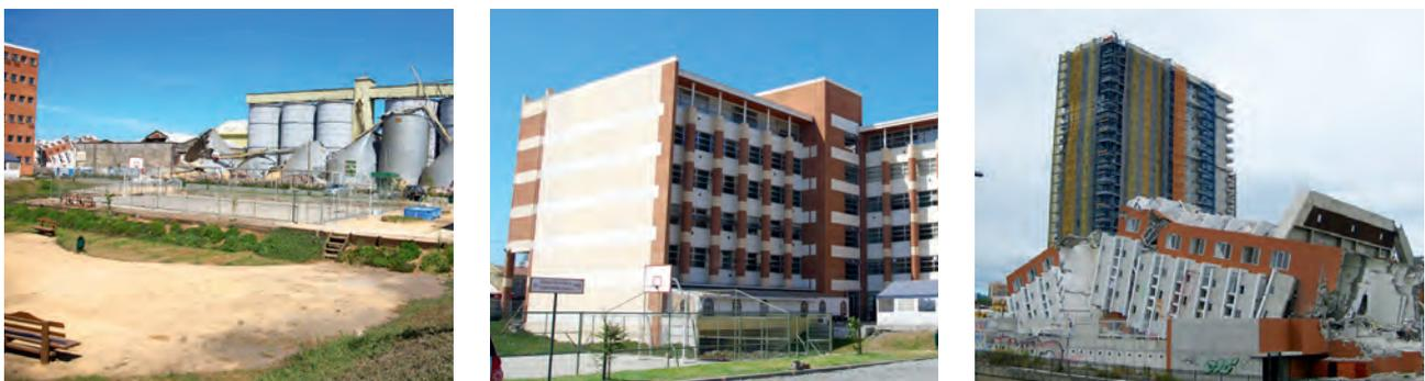
**Figure 10.** Three adjacent structures in Concepción, Chile are shown in the top photograph after the 2010 earthquake. The collapsed steel silos in the foreground of the first photograph are much newer than the much less damaged and much older steel silos in the back. The lightly damaged building in the left of the first photograph is shown in the middle photograph. It is much older than the collapse new tall apartment building in the third photograph. The collapsed building was new.
