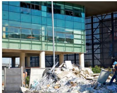
**Figure 3.** Damage to a transportation computer center inside an undamaged building in Concepción, Chile. Note the undamaged glass facade of the building. The third photograph shows a server room with inadequately braced/anchored and now destroyed servers, IT equipment cabinets, and other related equipment.
