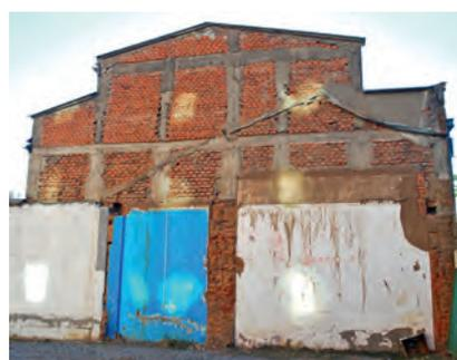
Figure 8. A lightly damaged confined masonry building in Talca, one of the most damaged cities of Chile in 2010.
