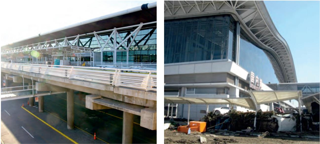
**Figure 9.** The new terminals at Santiago's International Airport (left) and Sendai's Airport (right). Both structures had light structural damage but extensive non-structural damage (and long business interruptions). Note the undamaged glass facades in both buildings. The lack of damage to the glass indicates that the structural design was excellent. The Sendai terminal suffered extensive tsunami damage to its first floor (the damage in the lower foreground).
