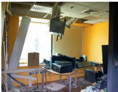
**Figure 2.** Structurally undamaged new concrete building in Santiago (upper left). Note the undamaged windows in the lobby and the water damage from broken water pipes in higher floors in the photograph on the upper right. The lower two photographs show interior damage to inadequately braced office partitions, suspended lights and other fixtures, suspended ceilings, suspended heating, air-conditioning and ventilating equipment, computers, etc.
