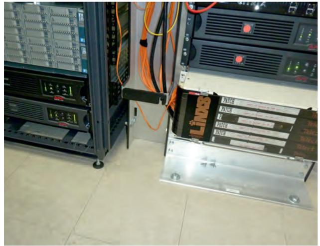
**Figure 5.** Unanchored and tipped-over electrical equipment in the 1999 M7.6 Central Taiwan earthquake. The solution (anchor bolts) is shown on the right of the right photograph. That particular IT rack is standing next to another one that is not anchored and that will fall over in a strong earthquake. The racks are part of the control system for a major Metro system in the U.S.
