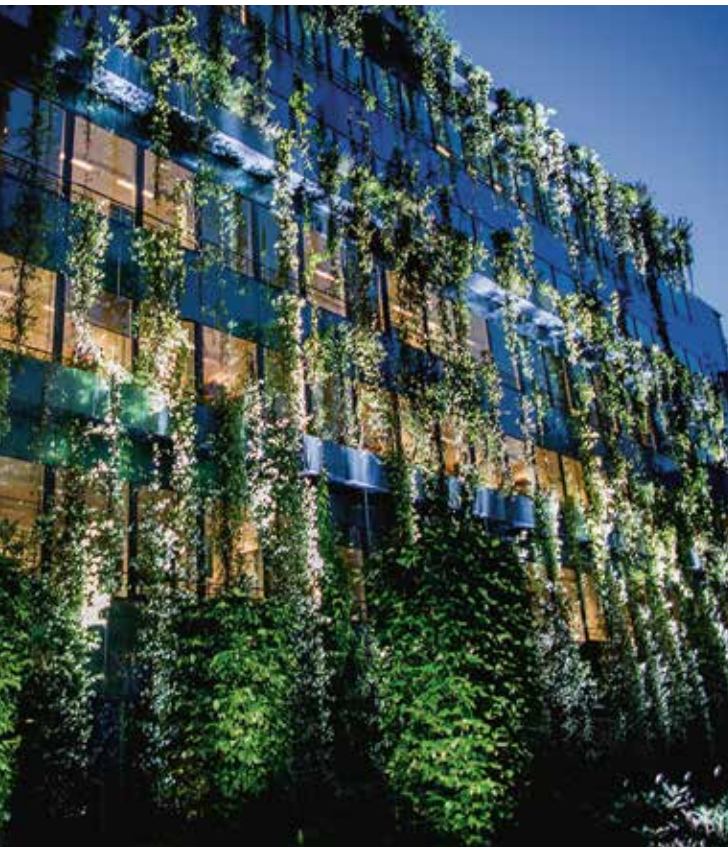
SCOR's Paris Headquarters, certified Haute Qualité Environnementale (high environmental quality) or HQE
