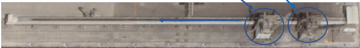
Unloaders sliding along the wharf and feeding the belt through a mobile roofing system
