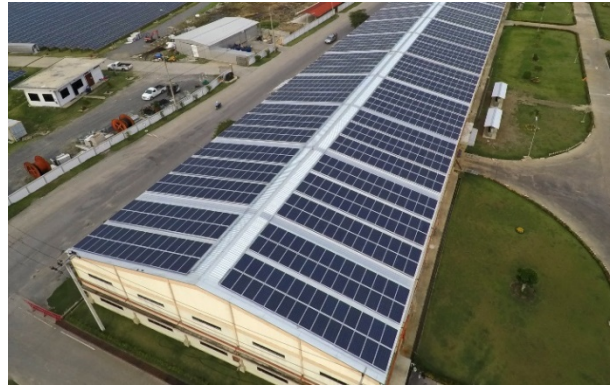
No air gap (not acceptable)
