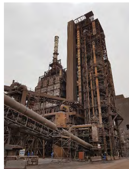
Process Gas Heater (left) DR Reactor (right)
