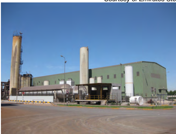
Air Separation Plant
