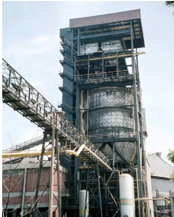
Coal Injection Storage & Conveyor to Blast Furnace
