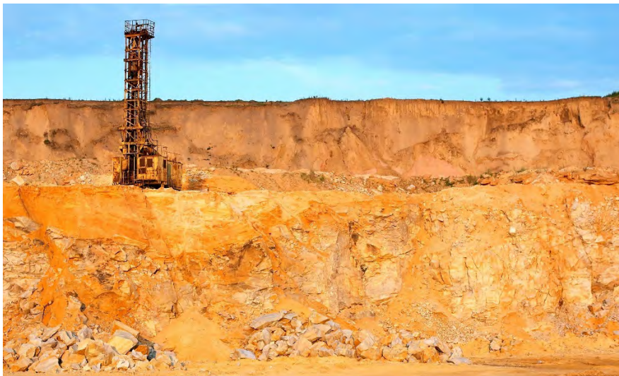
Drilling prior blasting
