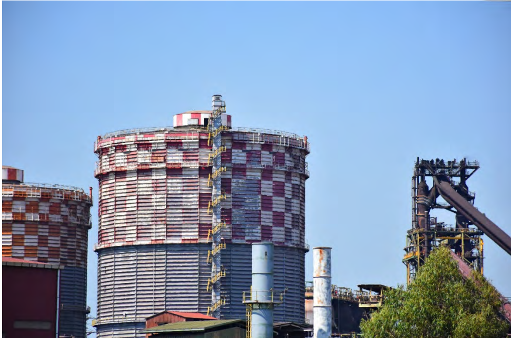
Coke gas pressurized tank
