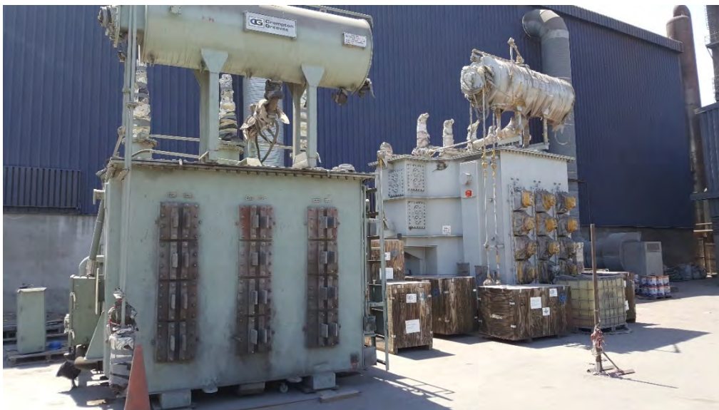
Spare AFTs for both EAF and LF Courtesy of Emirates Steel (ES) Abu Dhabi UAE
