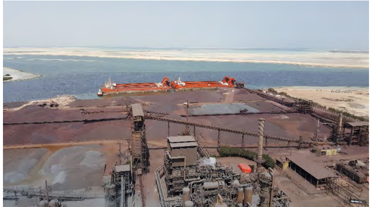
Wharf Courtesy of Emirates Steel (ES) Abu Dhabi UAE
