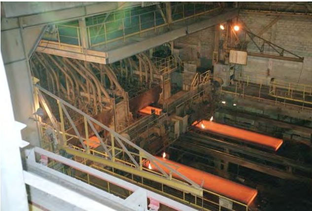
Slab Cutting Zone
