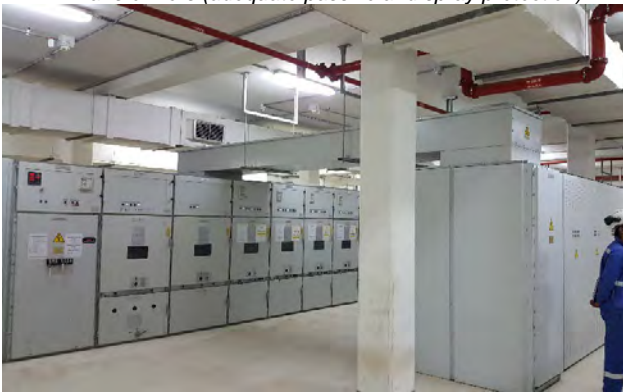
Integrated Steel Mill Main Substation (adequate total flooding FM200 protection)
