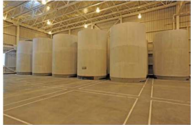
Source: Naval Nuclear Propulsion Program. Navy's spent nuclear fuel canisters surrounded by protective concrete overpacks in a storage building at DOE's Idaho site.
